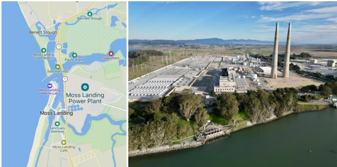
Located in Monterey County, California, the Moss Landing Power Plant has played a pivotal role in the state's energy landscape for decades. Construction began in 1949 under Pacific Gas & Electric (PG&E). By 1950, the plant was commercially operational with five natural gas and oil-fired steam units, delivering a combined capacity of 613 MW. Over the next 40 years, continued improvements and additions allowed Moss Landing to become California's largest power plant by capacity, reaching 2,560 MW.
