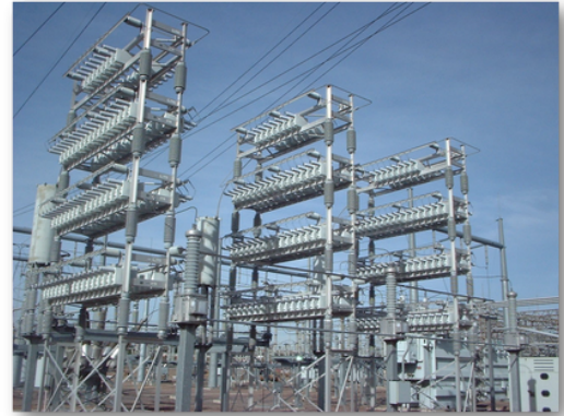
Substation Capacitor Bank
