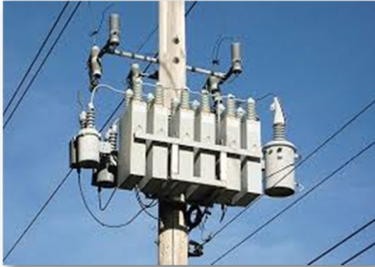
Distribution Switched Capacitor Bank
