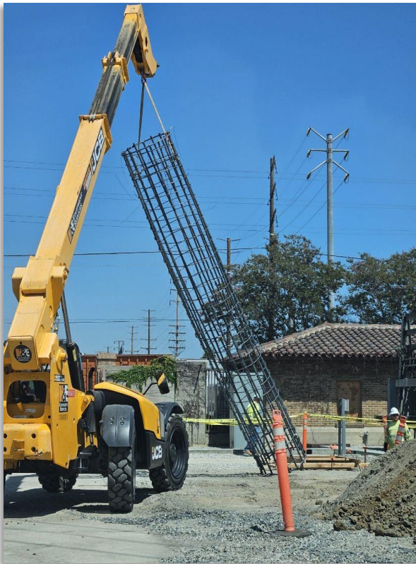
Steel Cage Install
