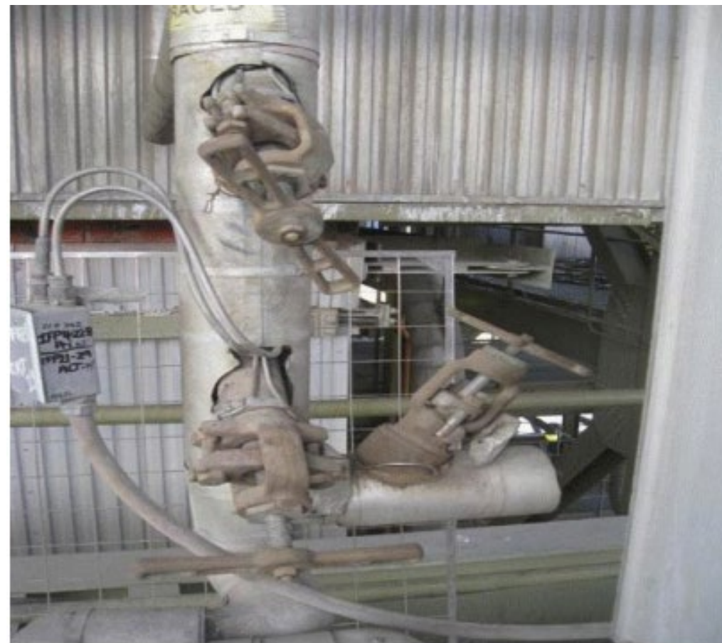
Exposed valves emerge from thermal insulation and are not heat traced.
