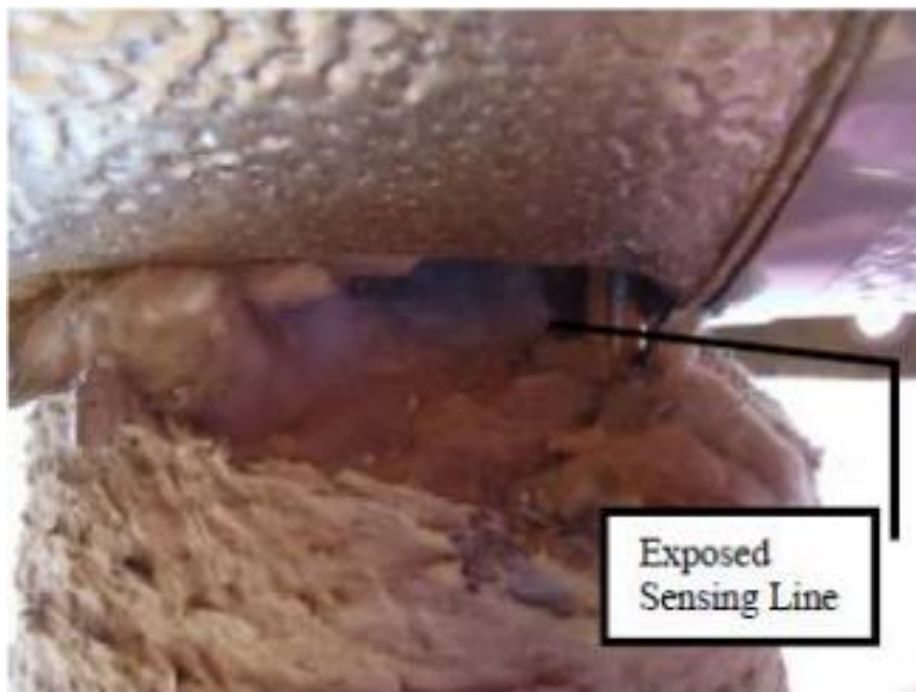
Gap in insulation
