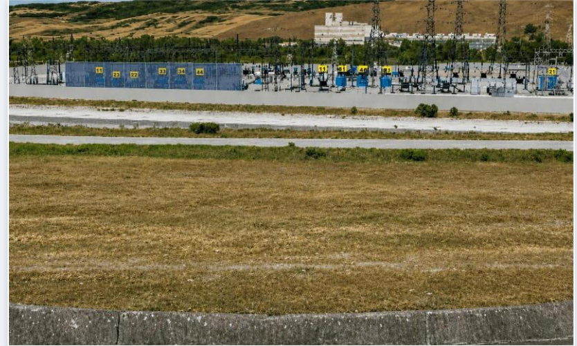
After — a ballistic steel barrier screens the bank's line of fire.
