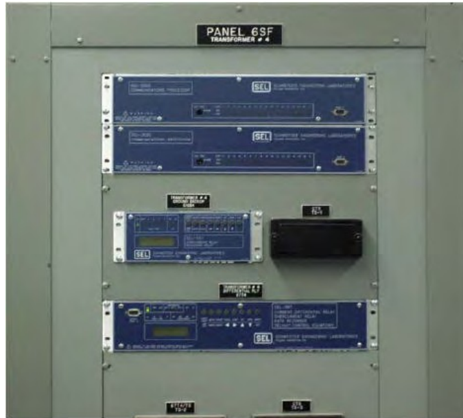
Figure 5.16b: Bottom half of Transformer Relay Panel
