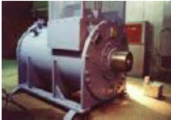
Figure 5.12: Synchronous Condenser
